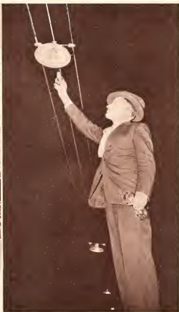
Changing infra-red globes used in the new type of citrus orchard heating is a simple matter. Sockets and reflectors are strung between the trees, as shown in this picture. Below: One light is used for every four trees, or forty lights to an acre. With the lights turned on, it is sufficiently light to permit night work.
